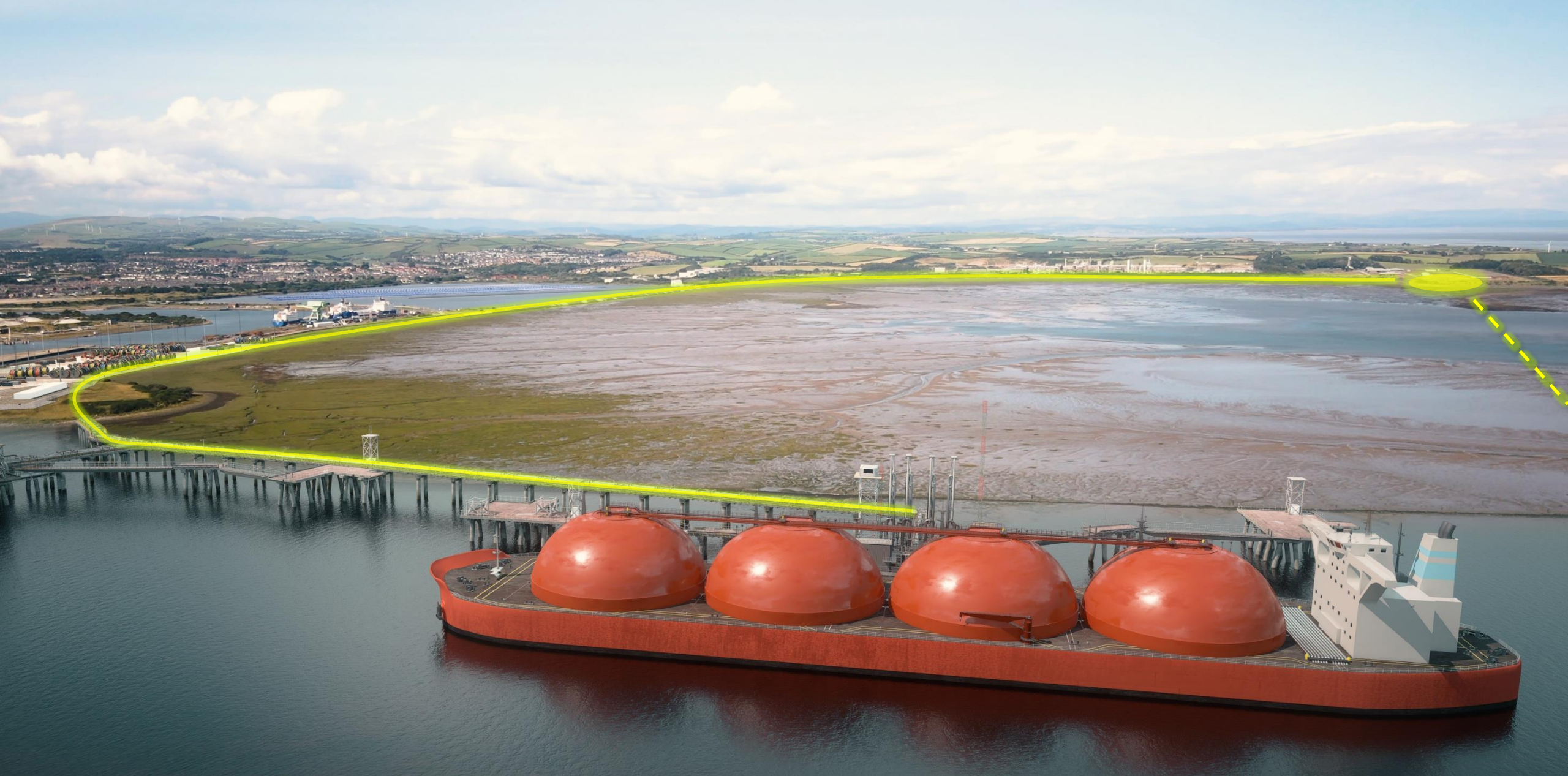
A new Walney Channel jetty for gas carrier vessels, with pipeline connection to the Spirit Rampside Gas Terminals
